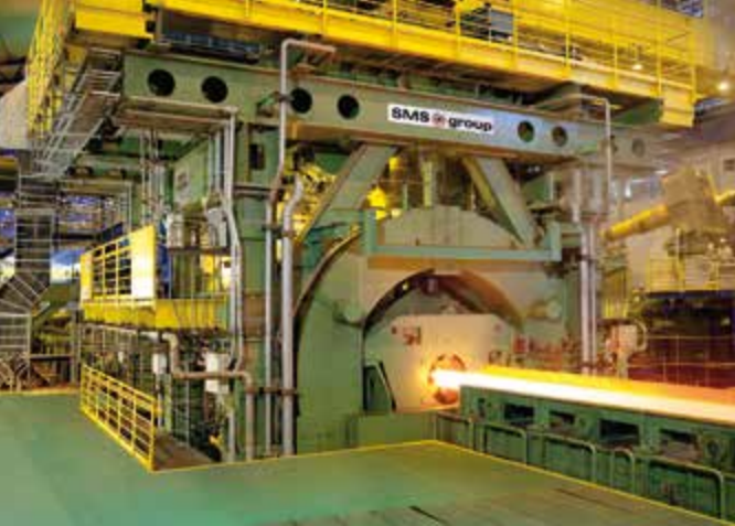
TUBE AND PIPE PLANTS
